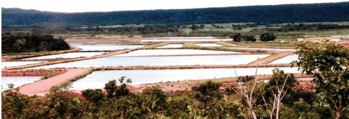
Piscicultura Princesa tanks, in construction in the Paraguay River headwaters region.
