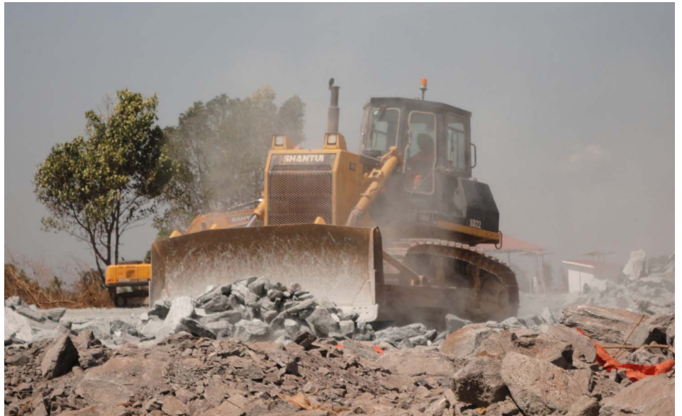
Demolition of houses in Awoo village. Photographer unknown.
