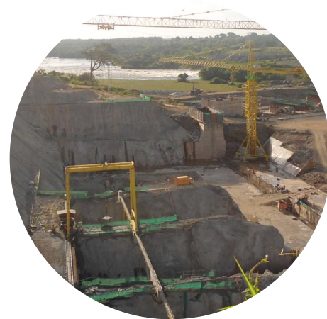
Karuma dam under construction. Photographer: unknown.
